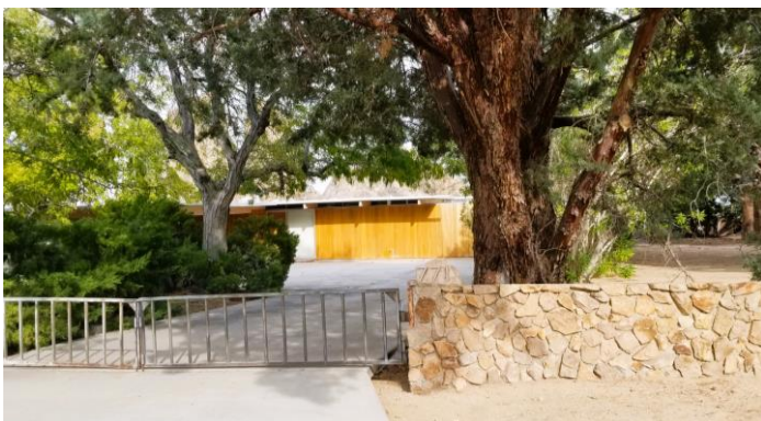
The street view of the Oyler House.
